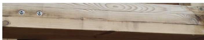
Surface delamination around glued edges caused by tension around knots.
