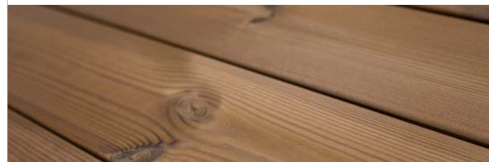
Unoiled Thermory Benchmark thermo-pine decking after installation
