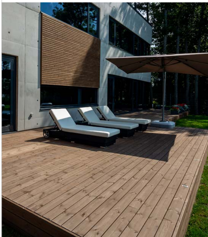
Oiled Thermory Benchmark thermo-pine decking Private house in Estonia Photo credits: Allan Leppikson
