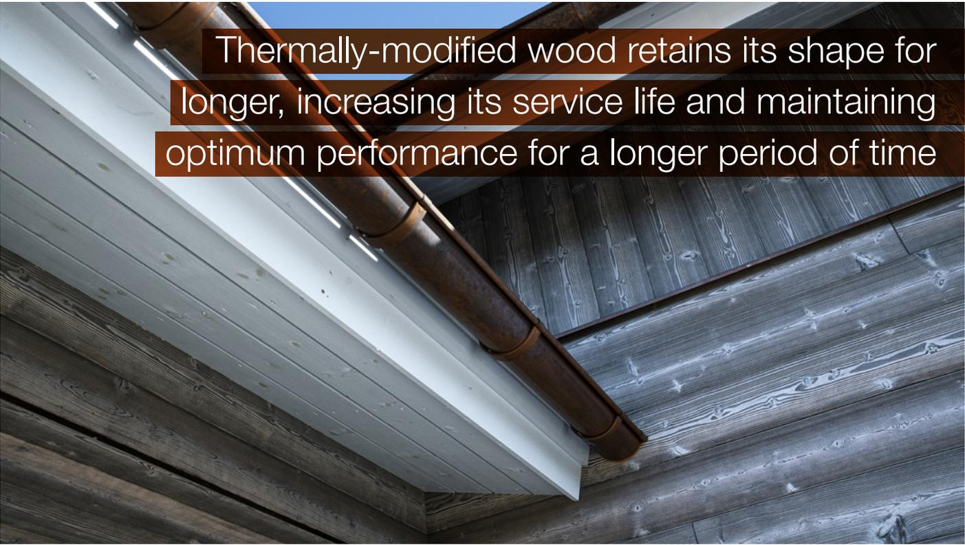
Thermally-modified wood retains its shape for longer, increasing its service life and maintaining optimum performance for a longer period of time
